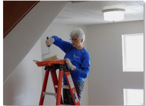
Above: Therese Sprunger painted the stairwell in March.
